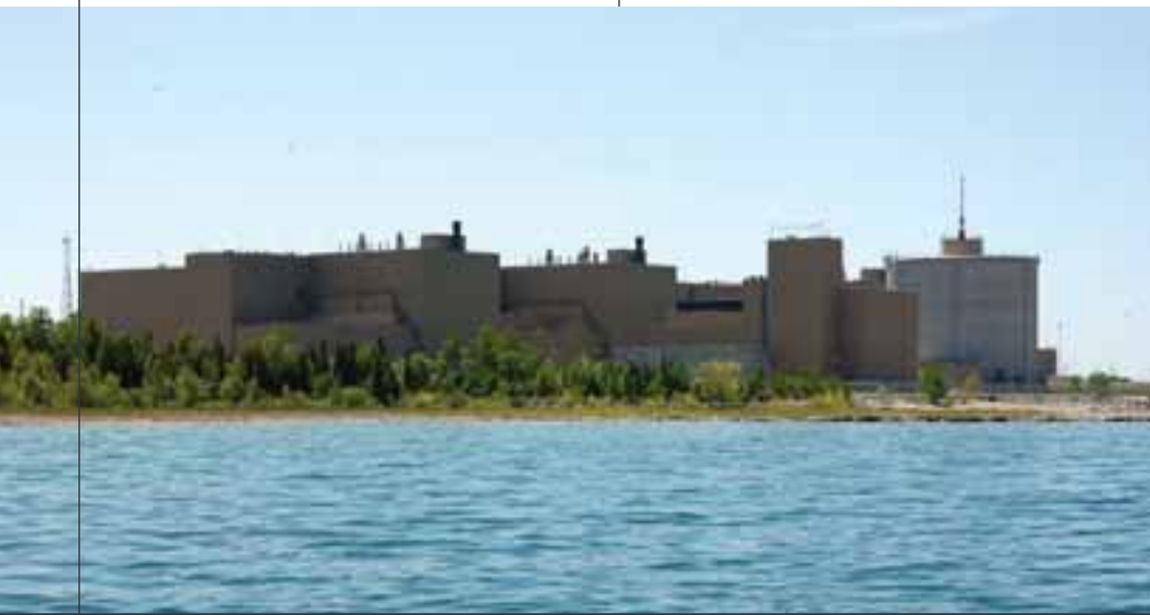
An exterior view of the Bruce B generating station.
