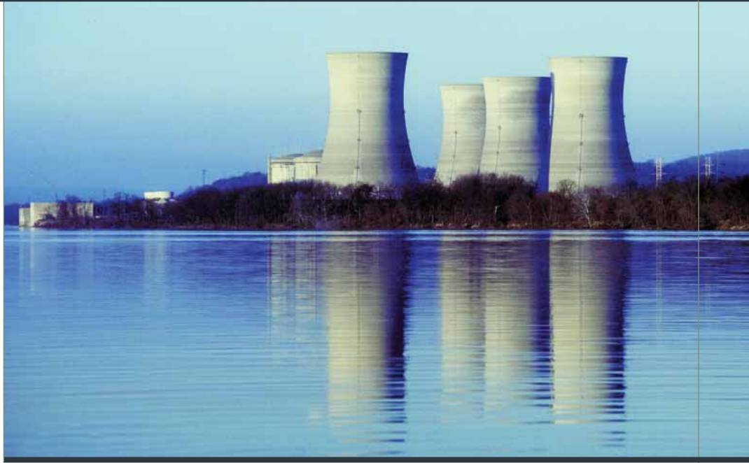
The facility at Three Mile Island.
