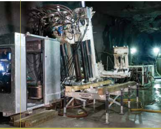
Raisebore Drilling at McArthur River Uranium Mine.
